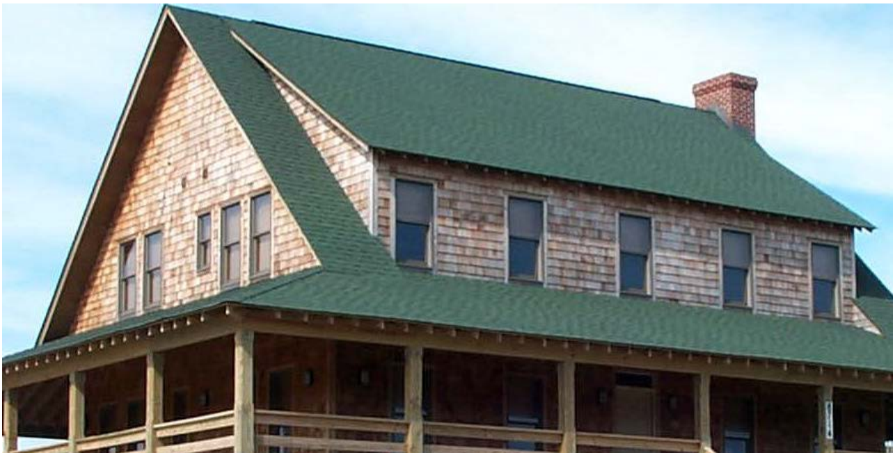
Wood Shingle Siding
