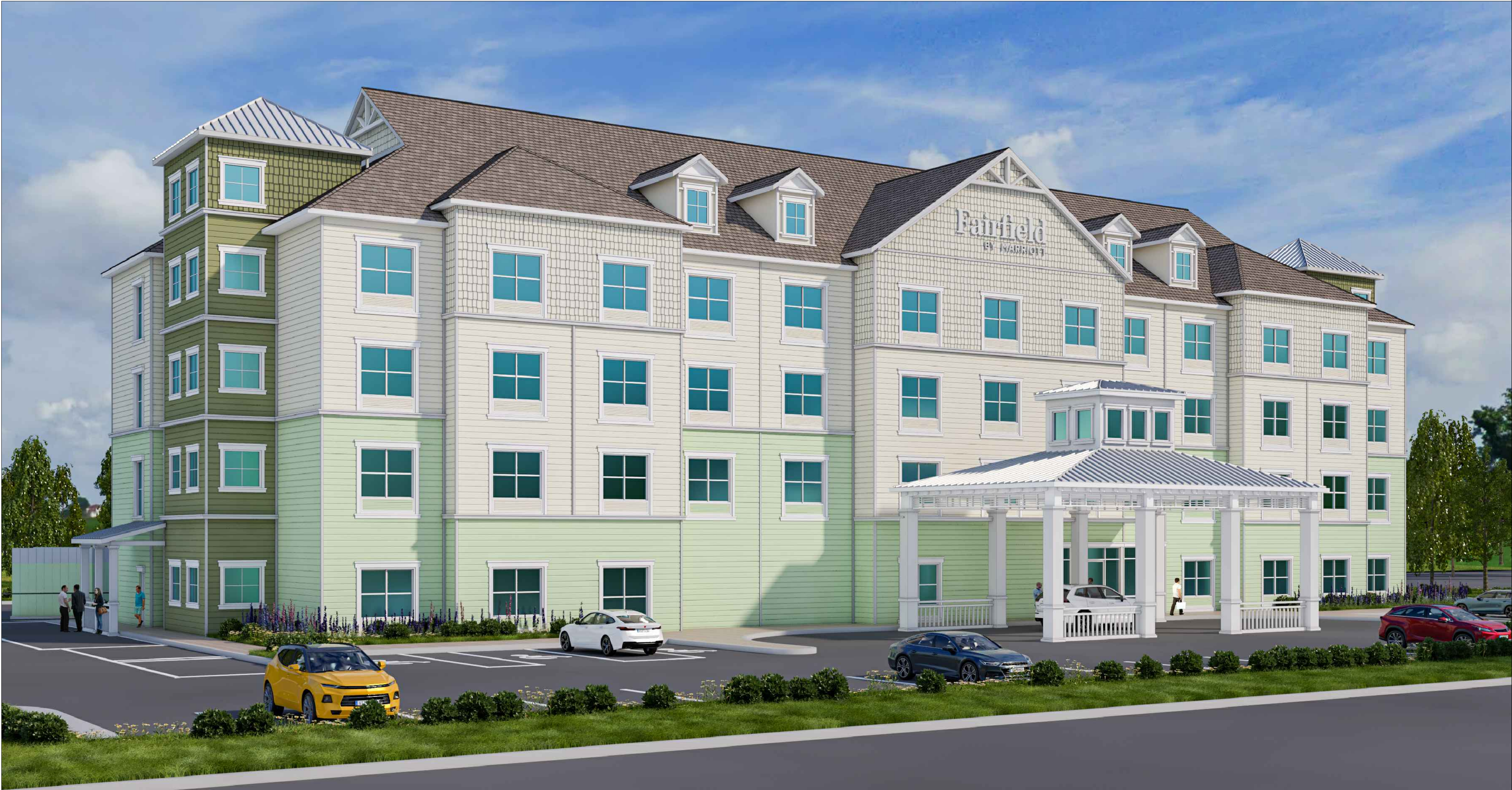
FRONT VIEW FROM SOUTH-EAST CORNER
